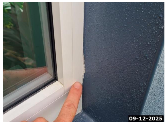
Damaged Paint / Sealant Around Window
