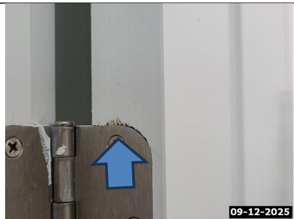
Sand Splintered Wood at Hinge Bore
