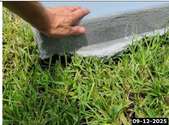
Gaps Under Slab – Ground Erosion
