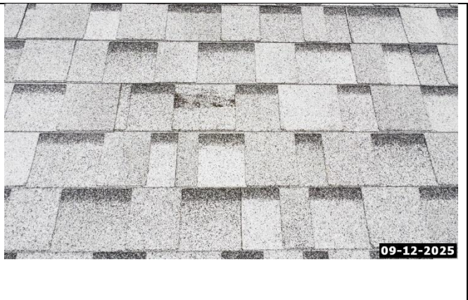
Damaged Shingle Visible
