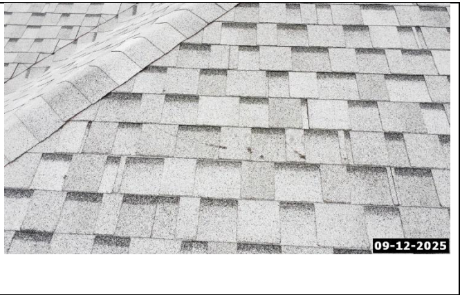
Damaged Shingle Visible
