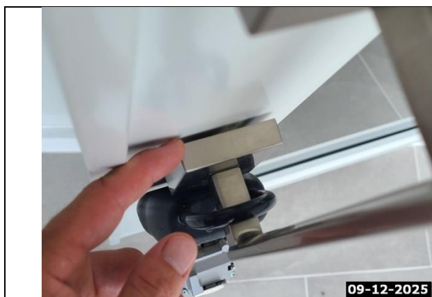
Bottom of Door Handle Not Secure
