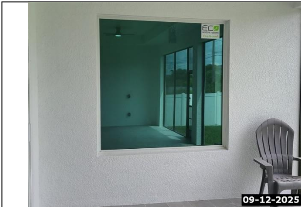
Caulking / Sealant at Window
