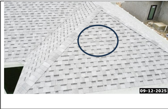
Damaged Shingle Visible
