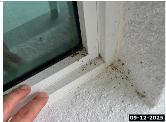
Caulking / Sealant at Window
