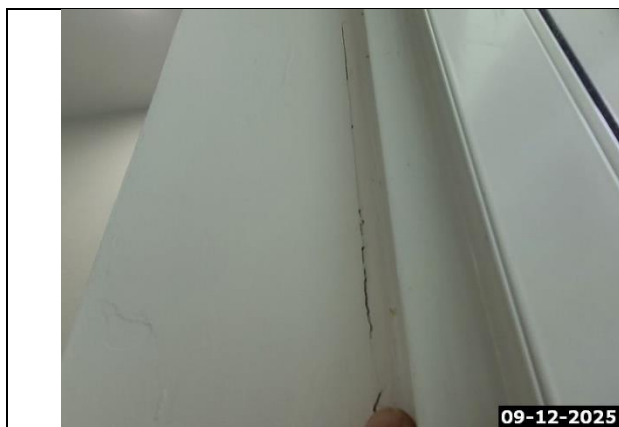
Cracking at Wall Around Door Frame at Exterior Door
