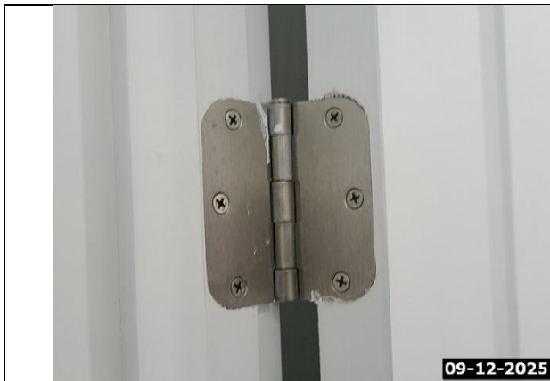
Sand Splintered Wood at Hinge Bore
