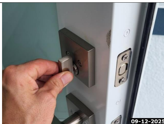
Movement at Deadbolt Turn Lever
