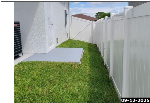
Slope at Sides of Home
