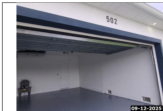
Trim Around Garage Door Opening
