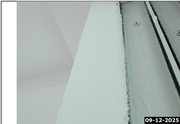
Joint Compound + Paint at Slider Components
