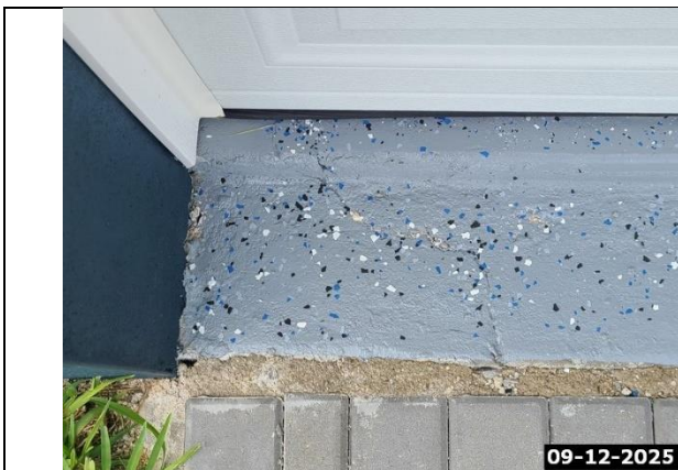
Crack Under Coating
