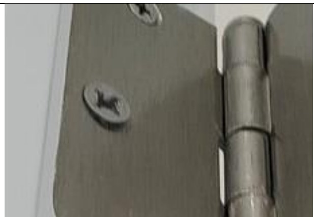
Door Hinge Hardware Misaligned (Master Bedroom Door)
