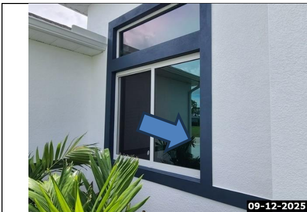
Damaged Paint / Sealant Around Window
