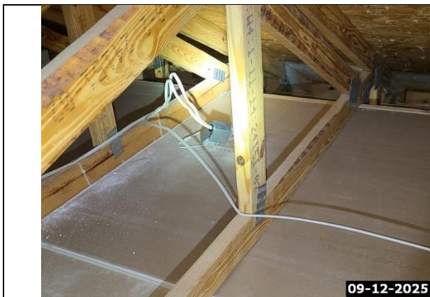
Recessed Light Fixture Hardware Not Secured In Place at Attic - All
