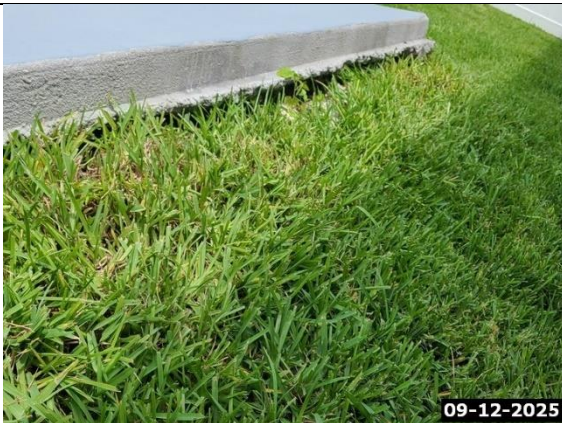
Gaps Under Slab – Ground Erosion
