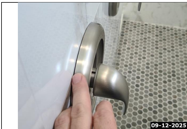
Shower Faucet Hardware – Install Caulk to Prevent Standing Moisture and Mildew Growth
