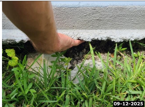
Gaps Under Slab – Ground Erosion
