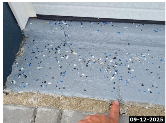
Crack Under Coating
