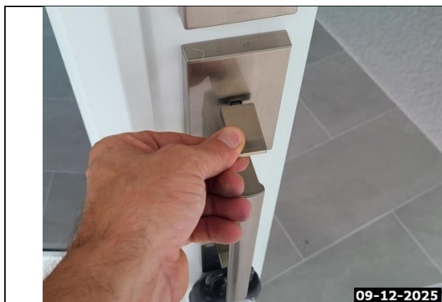
Movement at Door Latch Lever
