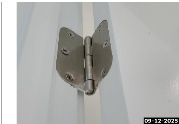
Paint at Door Hinge
