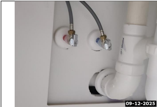
Bathroom #3 Sink Drain Gap In Wall Around Drain
