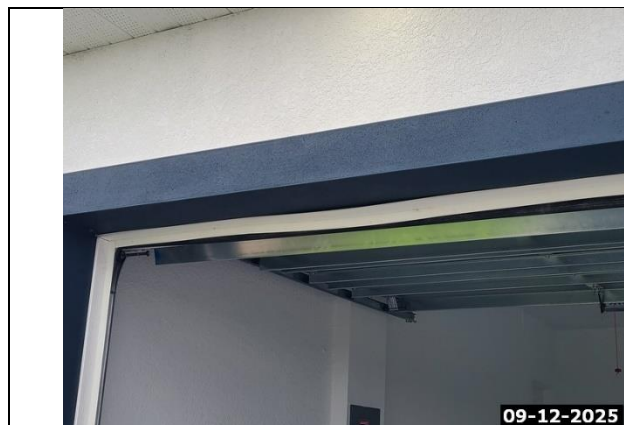
Trim Around Garage Door Opening
