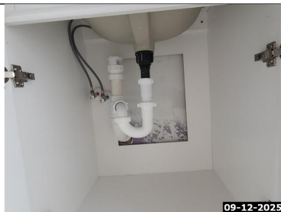
Bathroom #2 Sink Drain Gap In Wall Around Drain
