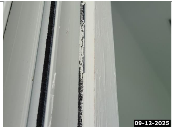
Joint Compound + Paint at Slider Components
