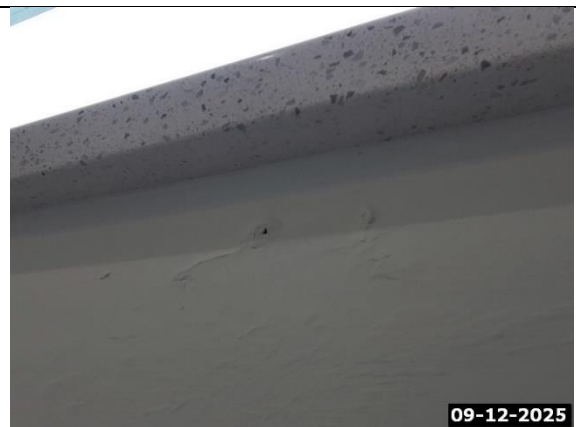
Screw Visible at Wall
