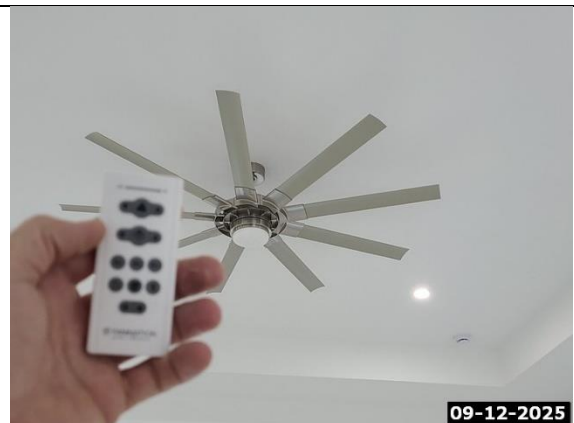
Living Room Fan Battery Dead
